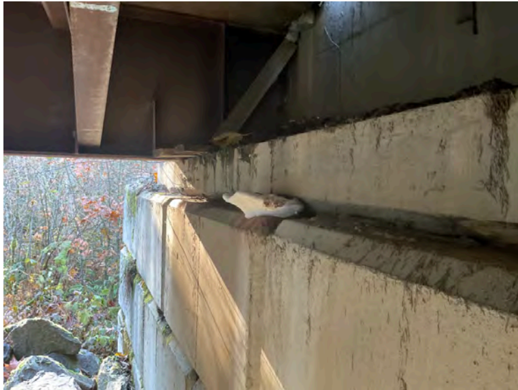
Fruiting body on left bank timber sill
