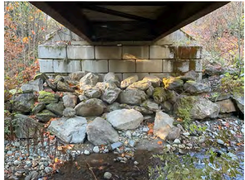
Right Bank Abutment when facing downstream
