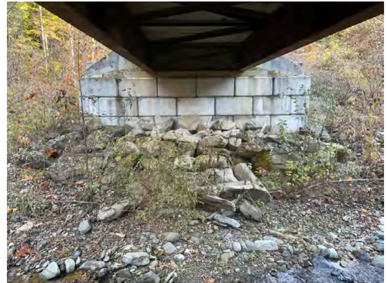
Left Bank Abutment when facing downstream
